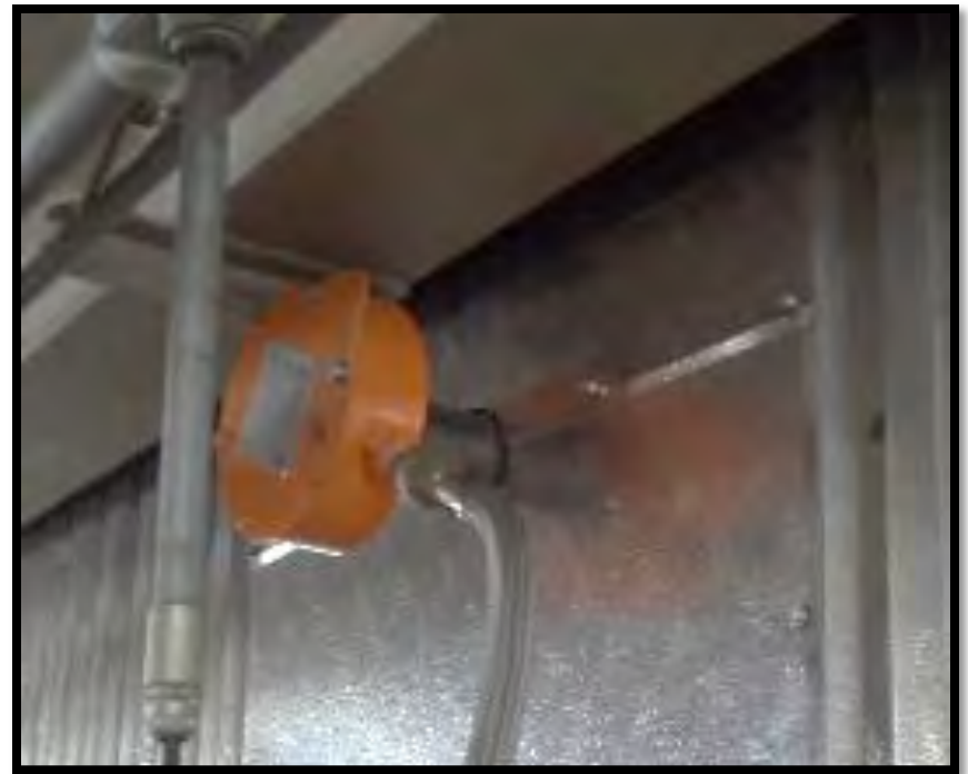
Model D-75 Retrofitted with Mega Sound Generator
